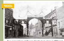
Two excavations of Bourne Castle took place in 1881 and 1889. The old castle gatehouse and part of the drawbridge were discovered. Bourne celebrated by erecting four grand archways within the town.
